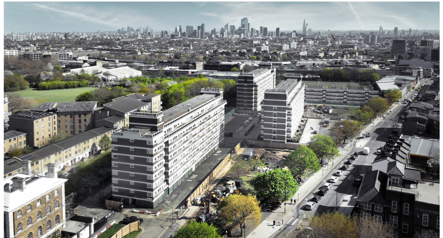
The York Way Estate sits on the former Metropolitan Cattle Market in London and includes four residential blocks
